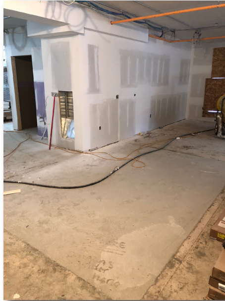
New slab. View from above shoring.
