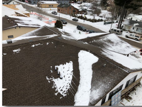
Aerial view of completed roof system.
