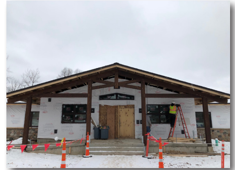
Front entrance timbers are complete.
