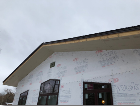
Soffit install is starting on the Southwest side.
