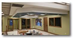
Circulation desk soffit is painted. The vertical face will be covered with custom fabricated wood veneer and trim.
