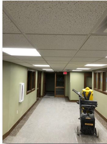
Ceiling tile is finished in lower level.
