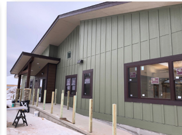
Overall look at the West side of the building.
