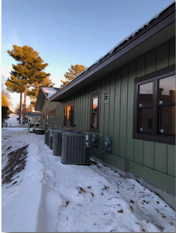
North siding is complete.
