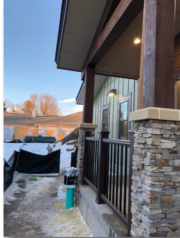
View of the West entrance canopy and railings.
