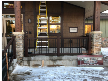
Trex Transend railings installed.
