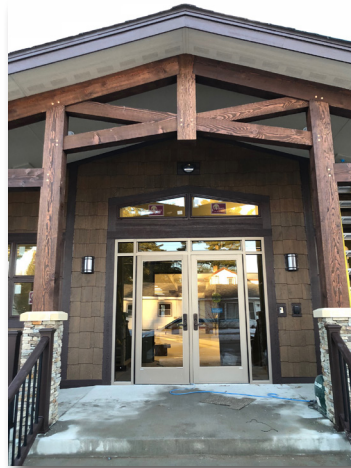
East entrance exterior is complete.
